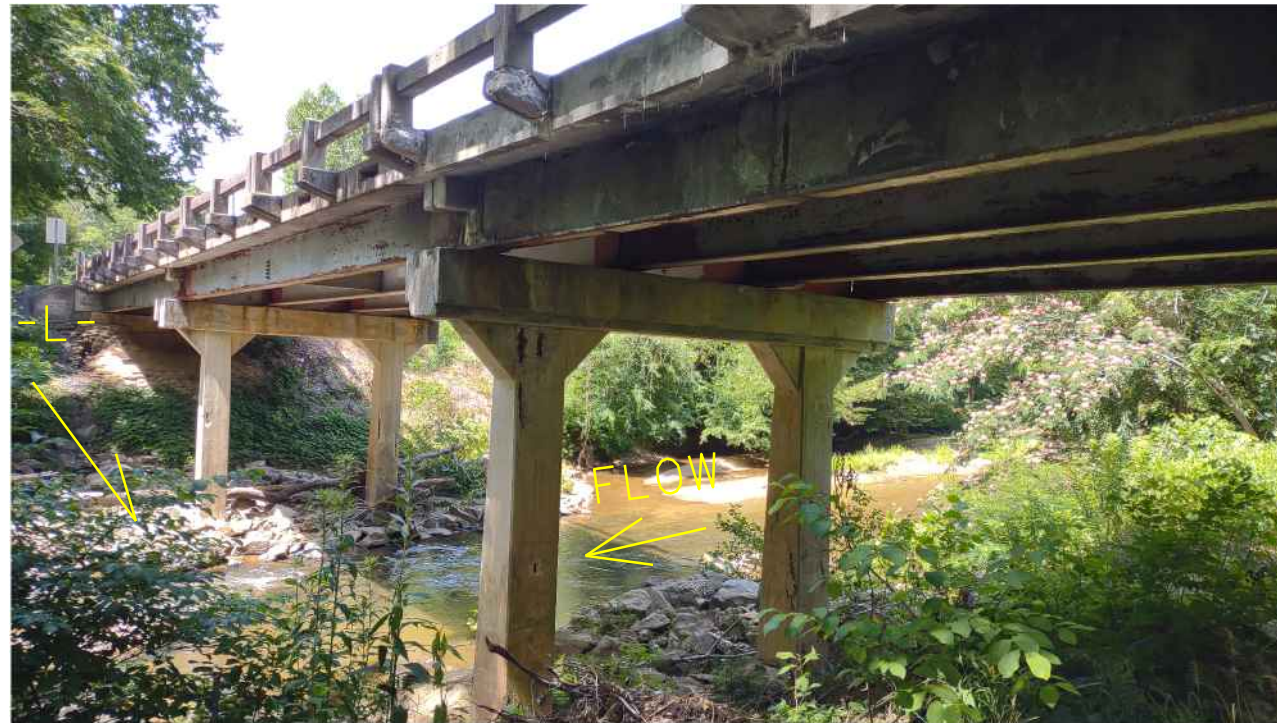
PHOTO #1: NORTH EAST SIDE OF EXISTING BRIDGE LOOKING WEST (DOWNSTATION)
